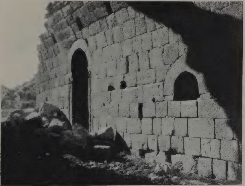
FIG. 170.—No. 43, door and niche, in monastery.
